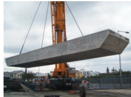
Breakwaters Unit with GRC Bottom Skin providing protection to the polystyrene floatation units.
